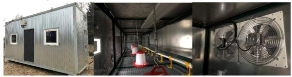
Fig. 2. Technological module for broiler fattening
